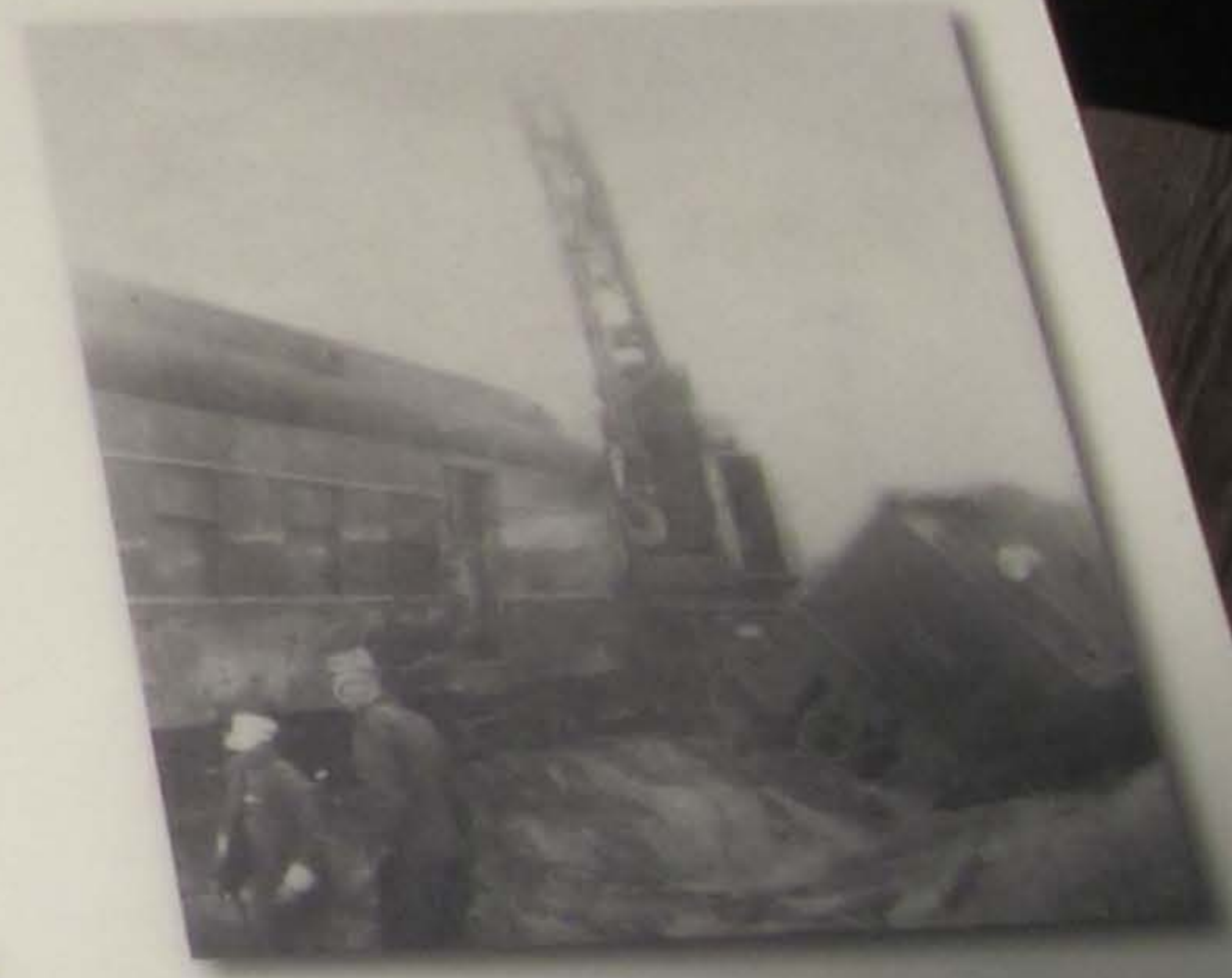
Below: Setting derailed cars back on the rail tracks
